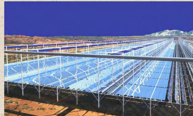
CHP linear Fresnel
