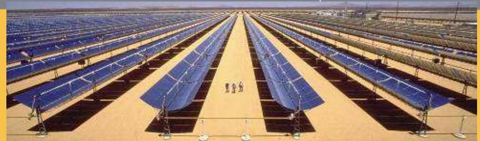
Linear parabolic reflectors
