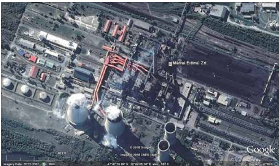
Fig. 4. Second type of plume merge in the Mátra Power Plant, Hungary.
